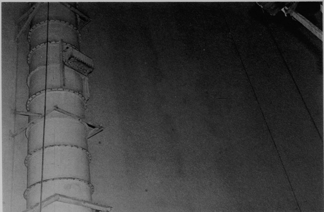
Figure 271 (6A). Ventilation duct on the containment wall, southwest quadrant.
