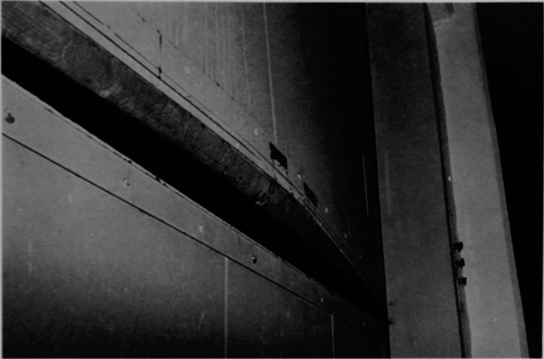
Figure 109 (6A). Close-up of gap in elevator door (elevation 347).
