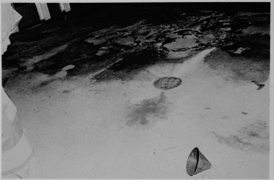
Figure 19 (1A). Floor drain and rusted funnel (center detail of Figure 18).
