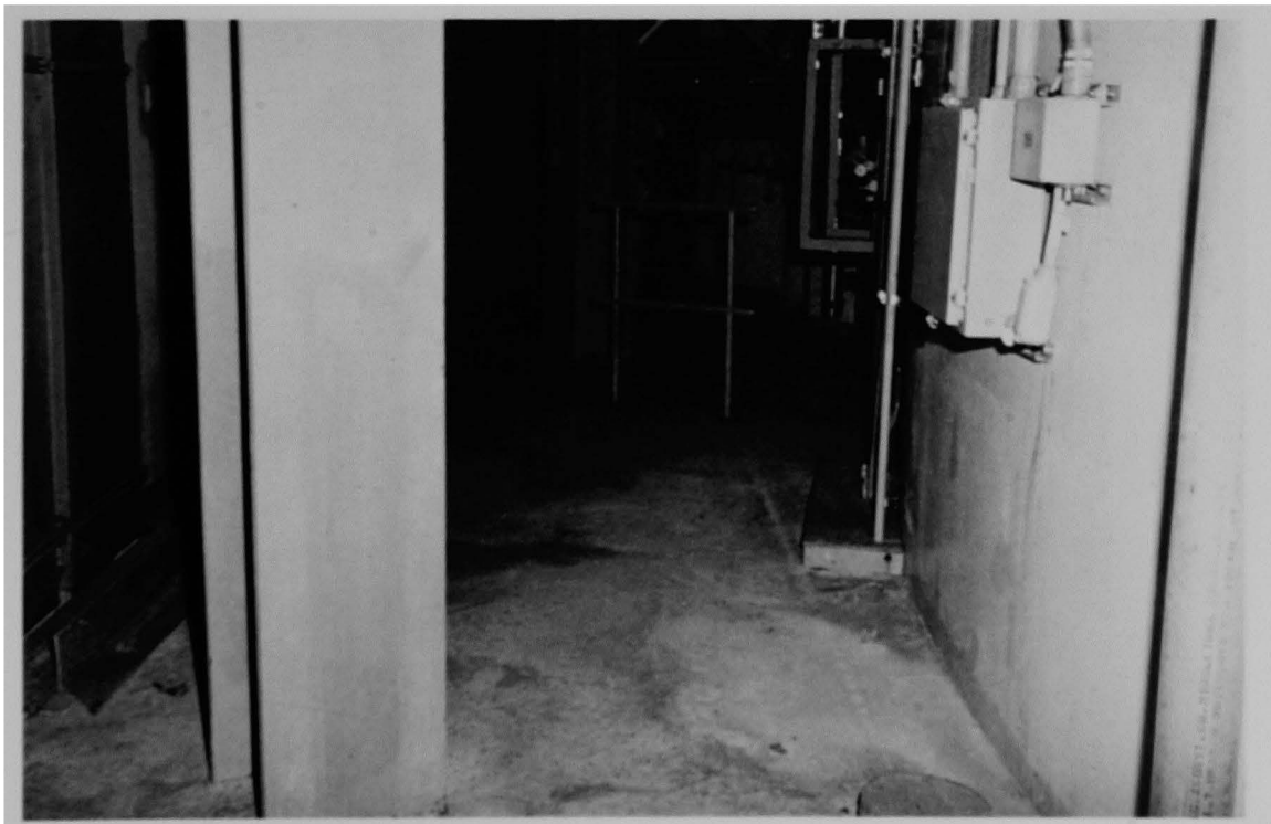
Figure 71 (5A). Northeast view taken north of open stairway; wall shielding incore instrumentation cable chase in background.
