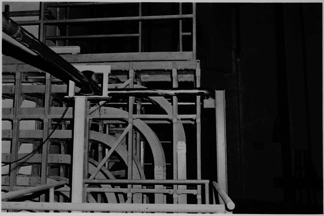
Figure 100 (2A). Control rod drive mechanism cable trays (see Figure 97, left).
