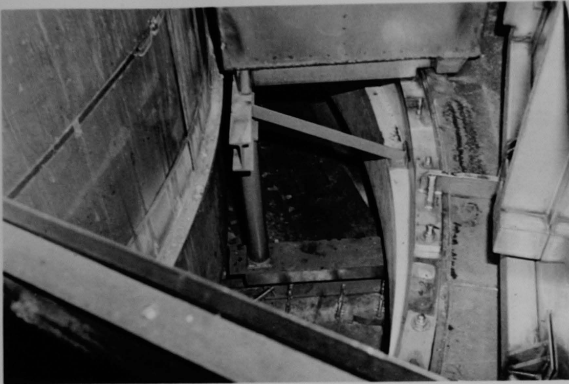
Figure 257 (5A). View underneath a neutron shield tank.
