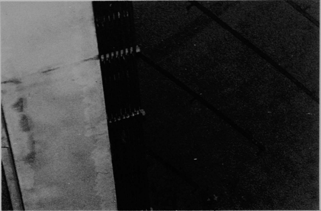
Figure 306 (5B). Trolley power and controller buss bars, view from the midpoint of the polar crane access ladder.
