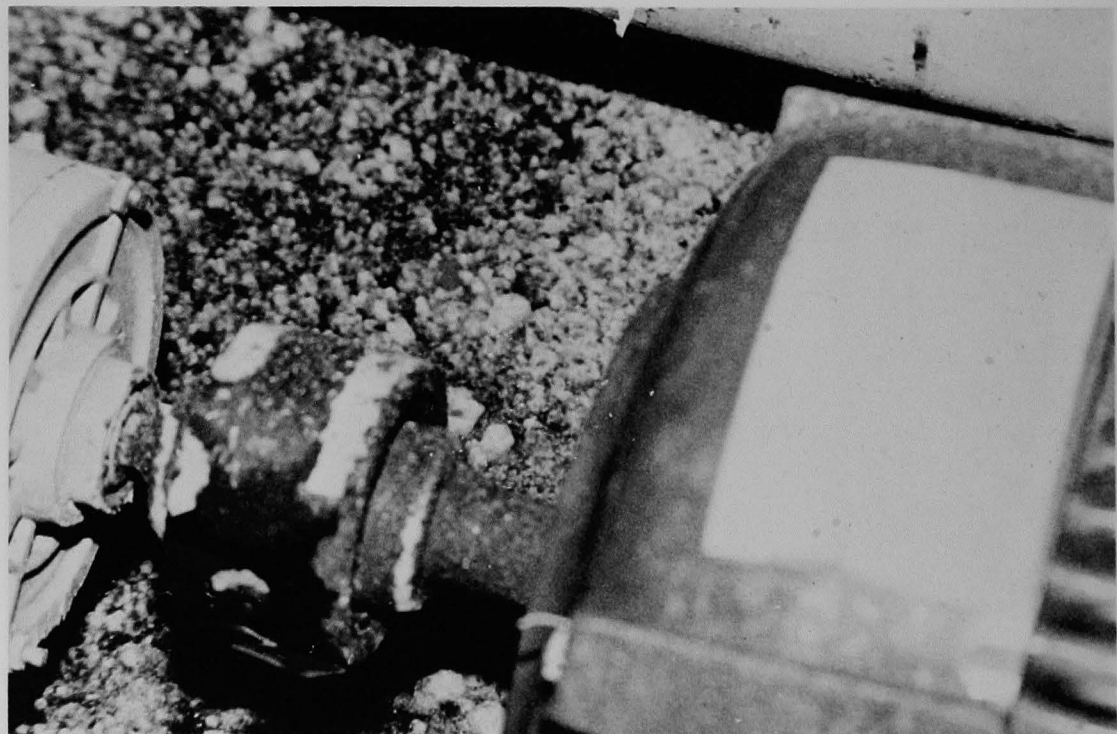
Figure 224 (5B). Rusted coupling and motor on auxiliary fuel handling bridge (see Figure 222).
