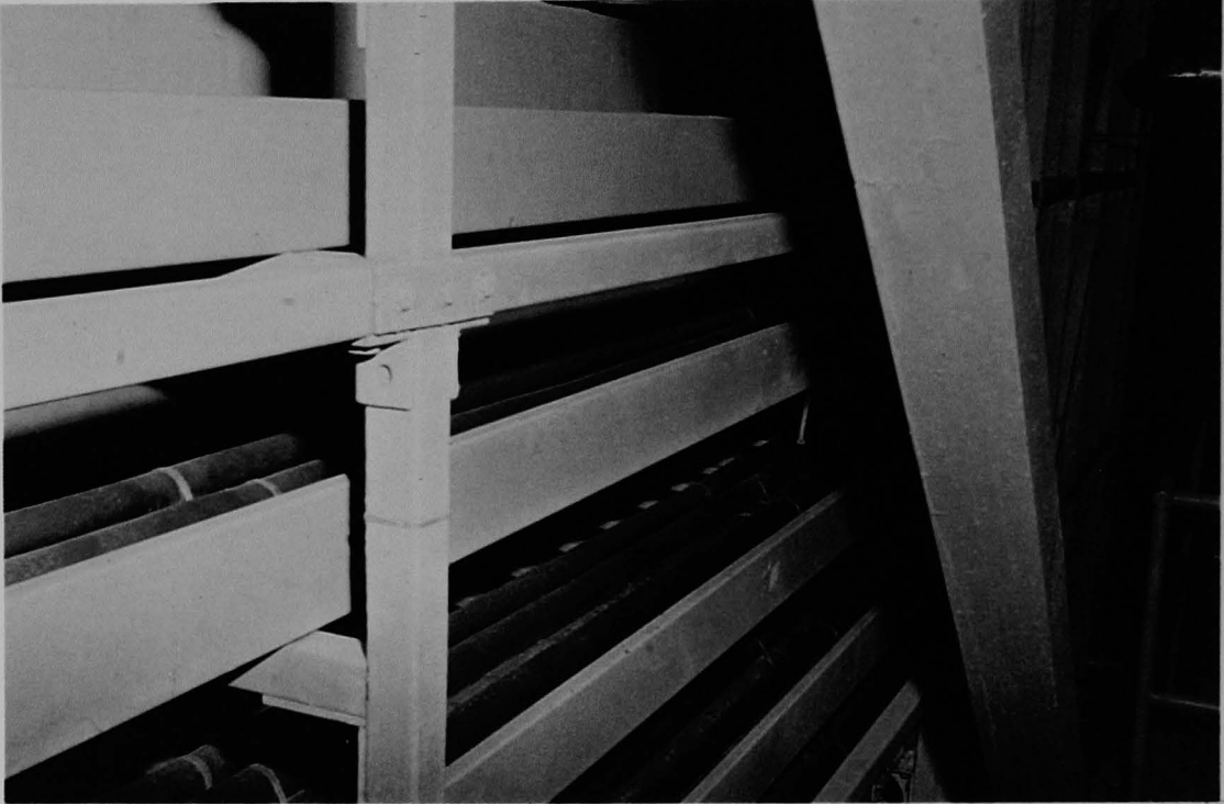
Figure 251 (6A). Close view of CRDM cable trays; hand rail to auxiliary fuel handling bridge right.
