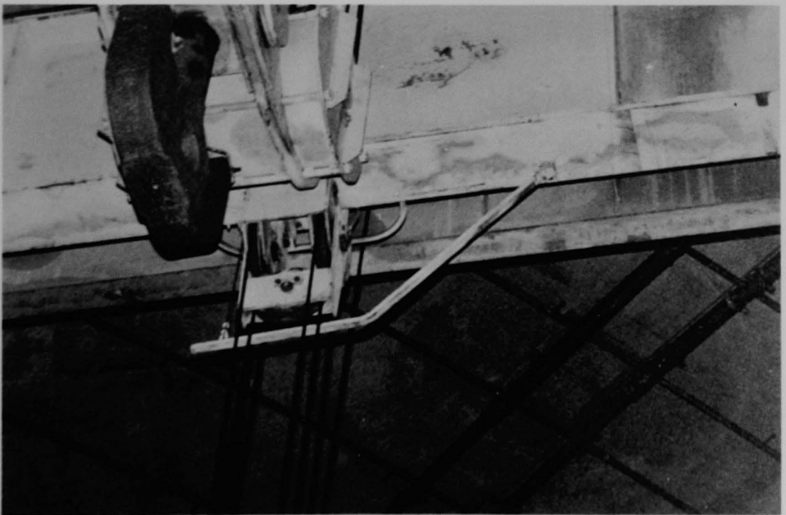
Figure 293 (5B). Main hook of the polar crane, second view.
