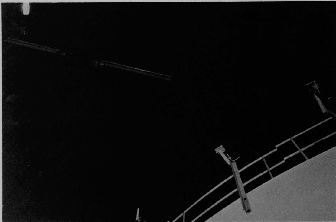
Figure 286 (2B). Jib crane and support box, southwest quadrant.
