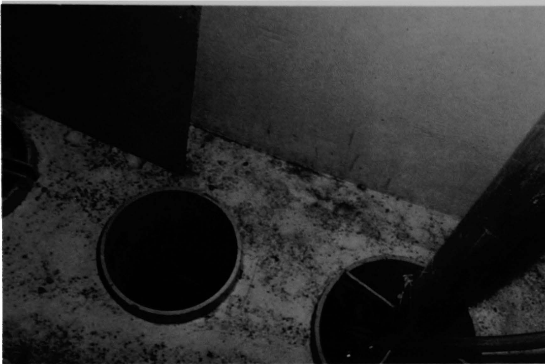
Figure 82 (6A). Floor penetrations 211 and 212 (cf. Figure 81).
