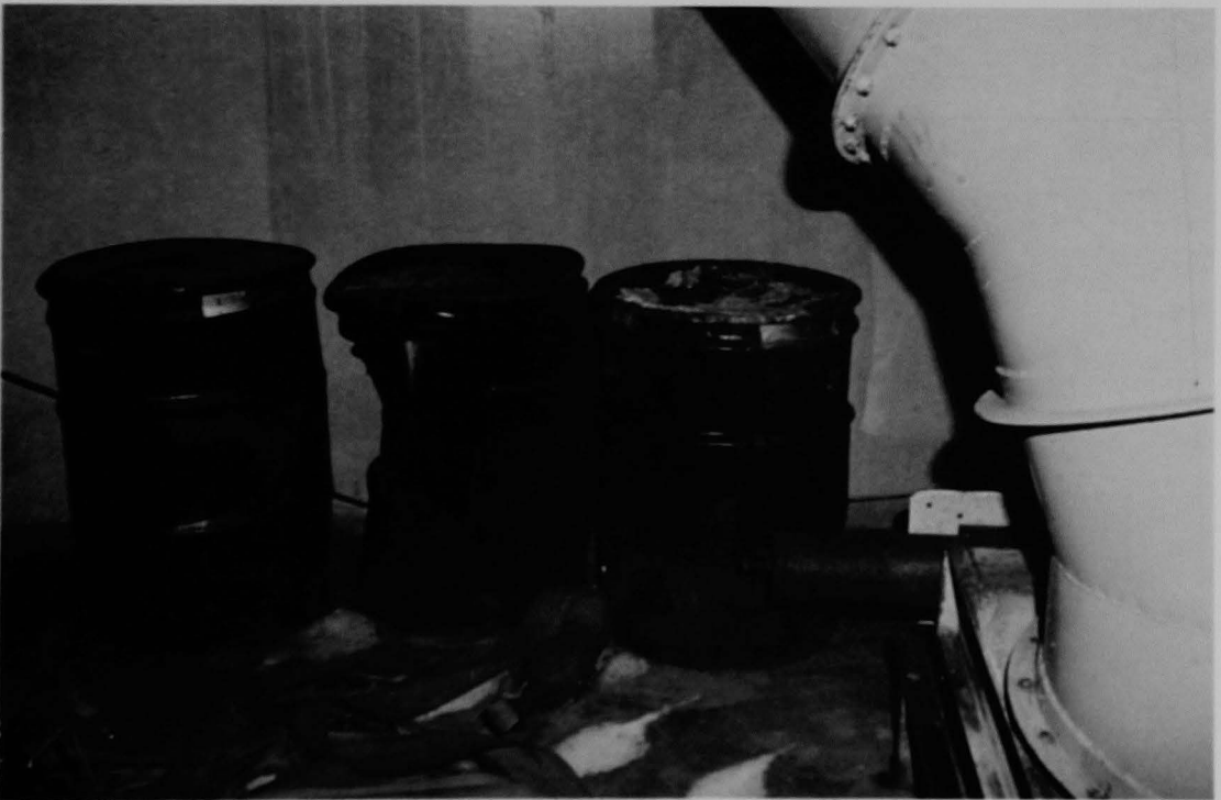
Figure 122 (4A). Fifty-five gallon drums between enclosed stairwell and air duct.
