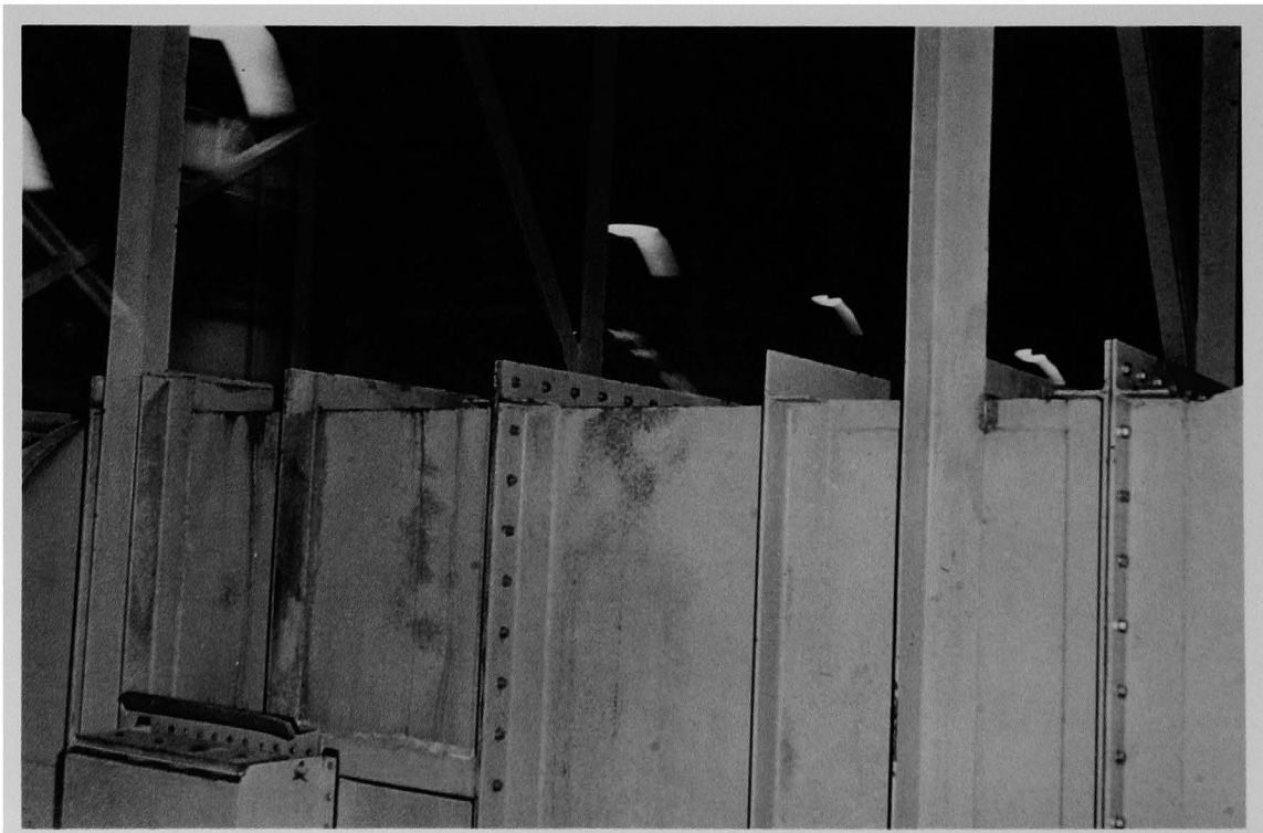
Figure 32 (6A). Portion of top section of the air coolers, view from platform on enclosed stairwell.
