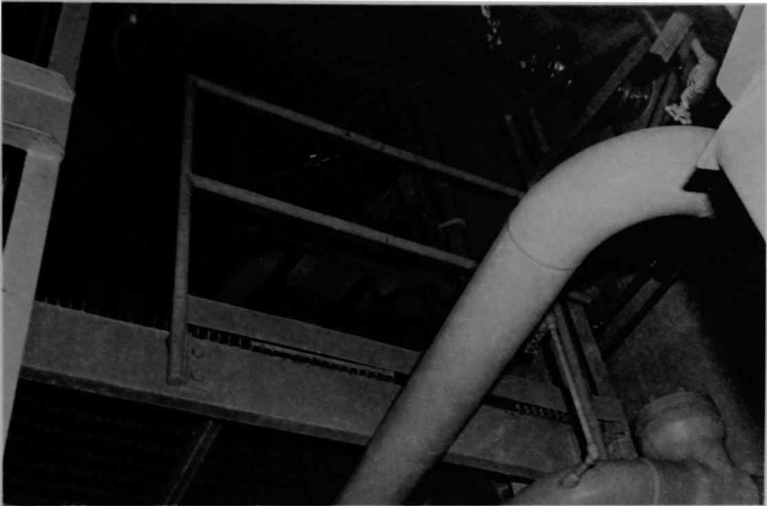
Figure 86 (6A). View up to the overhead piping, grating, and cables near core flood tank A.
