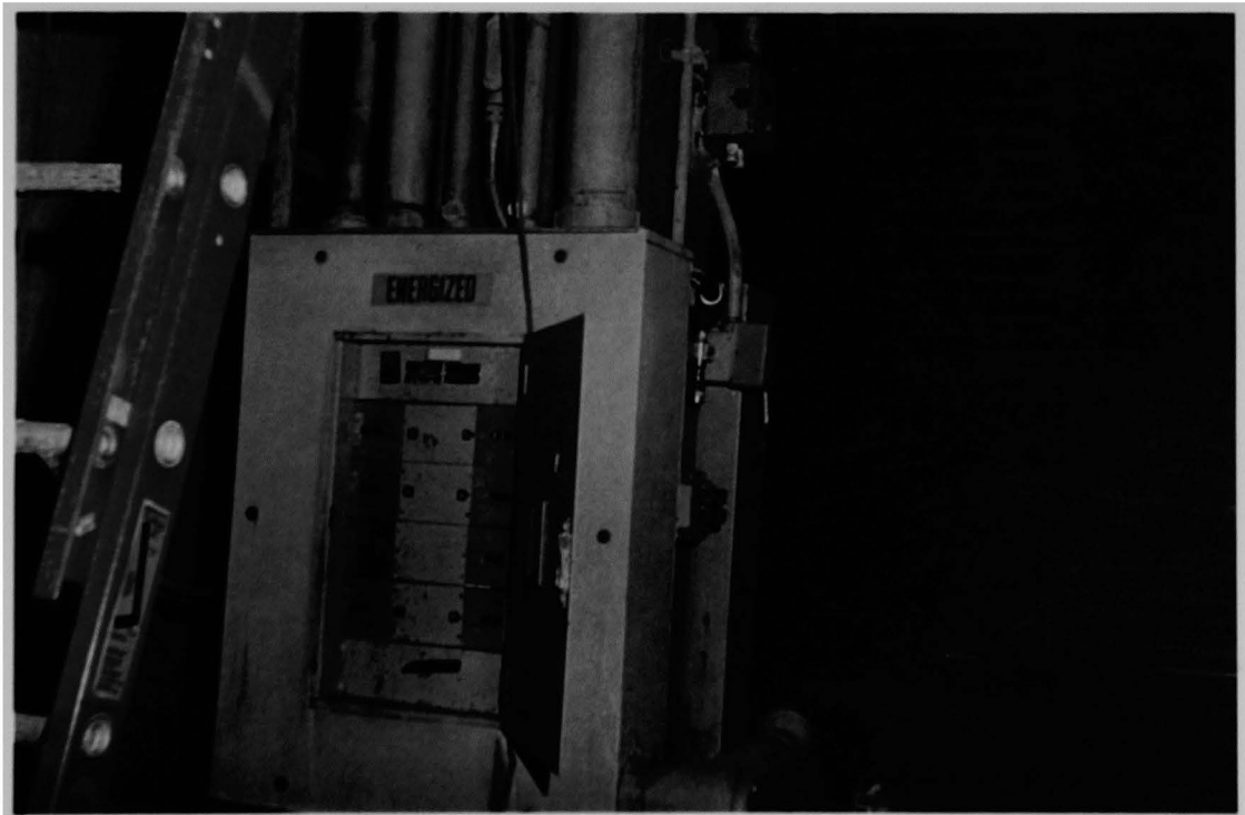
Figure 53 (2A). Power panel on I beam; open stairway in background.
