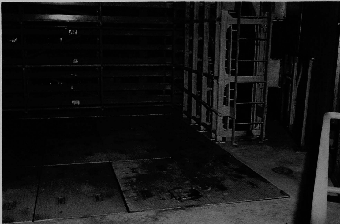
Figure 194 (4A). Decking over core flood tank A; cable trays background.
