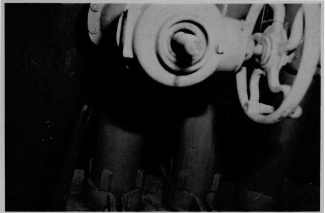
Figure 25 (2A). Bottom corner of door to enclosed stairwell, thrust against structure of river water piping.
