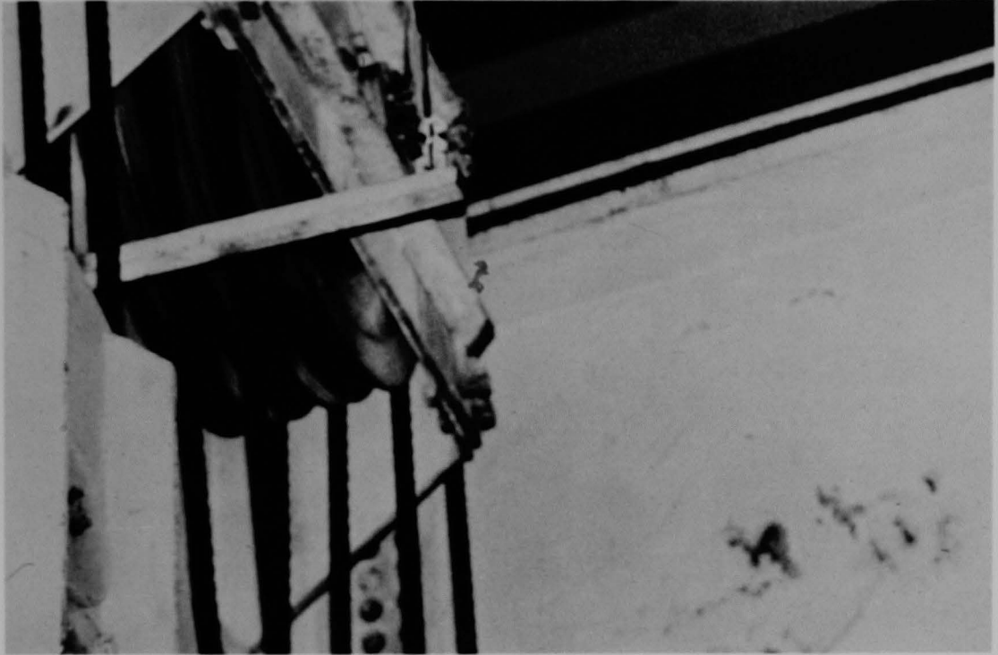
Figure 300 (5B). Close-up of cables for the main hook.
