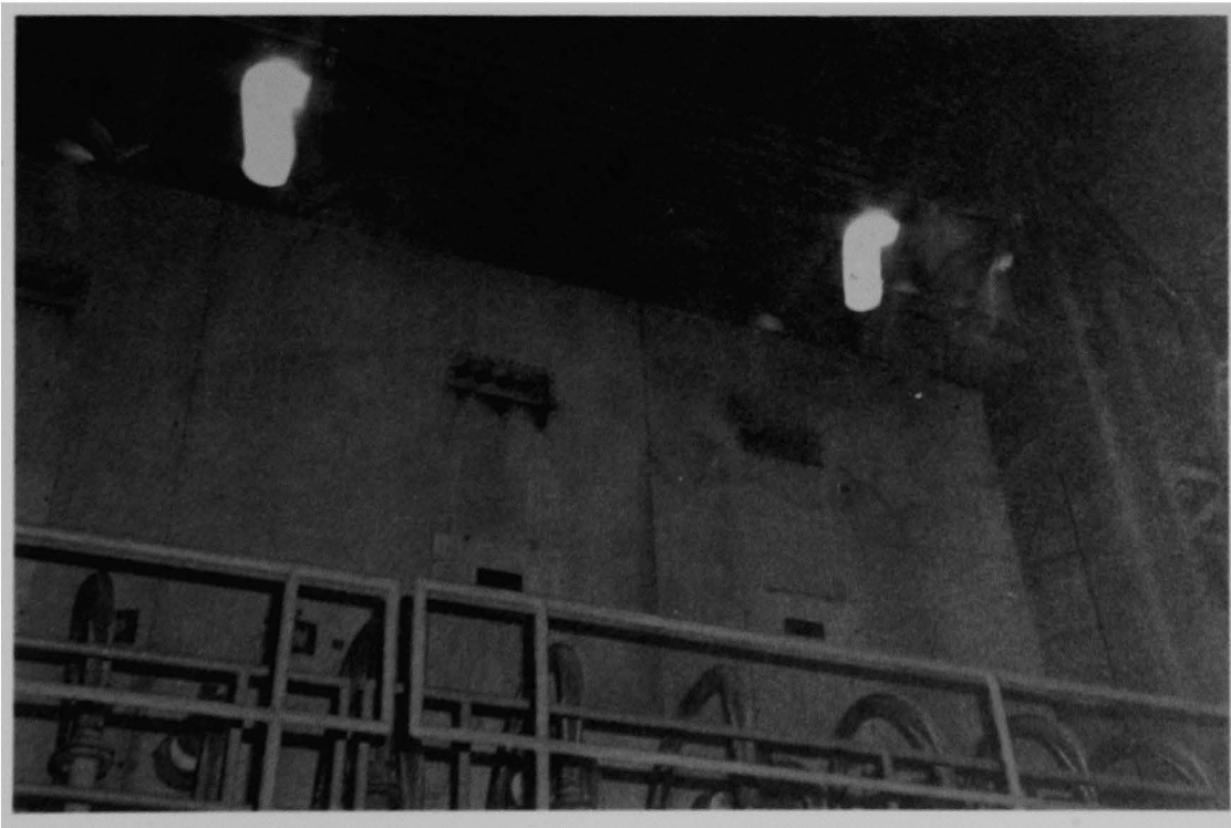
Figure 45 (6A). West upper end of air cooling assembly.
