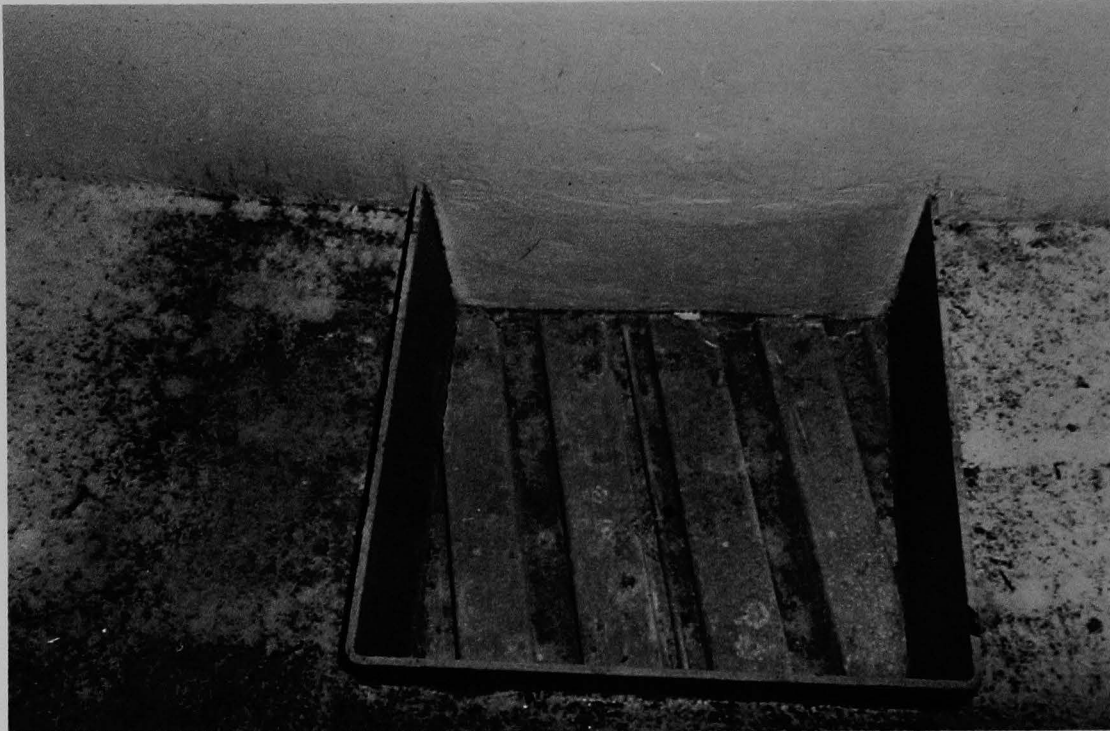
Figure 190 (5A). Floor penetration 266, along east side of D-ring wall.
