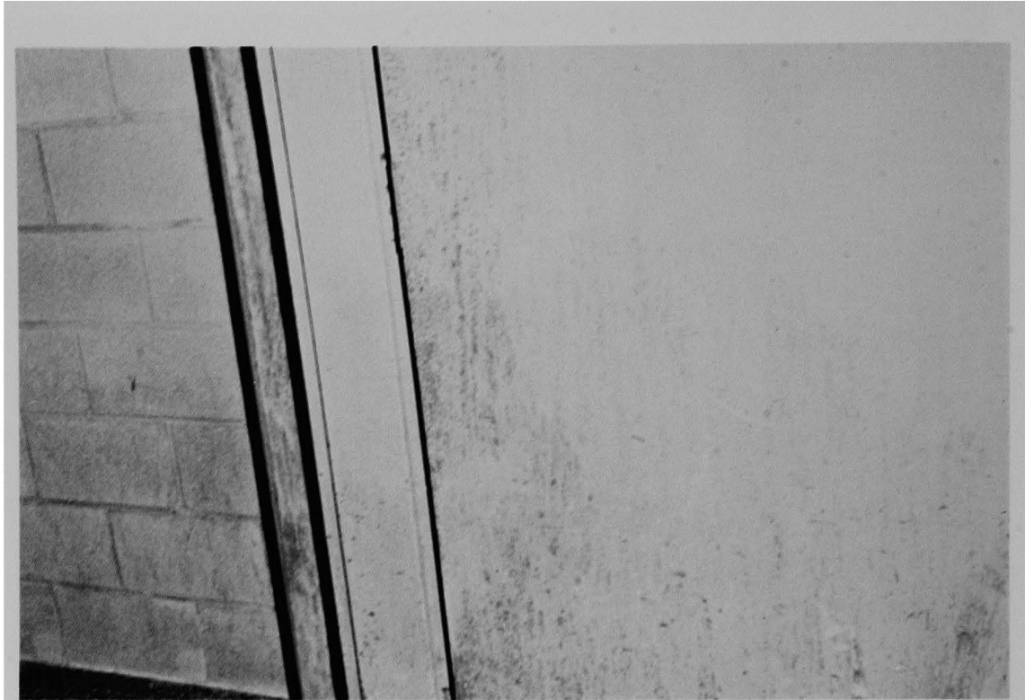
Figure 27 (1A). Surface of door to enclosed stairway.
