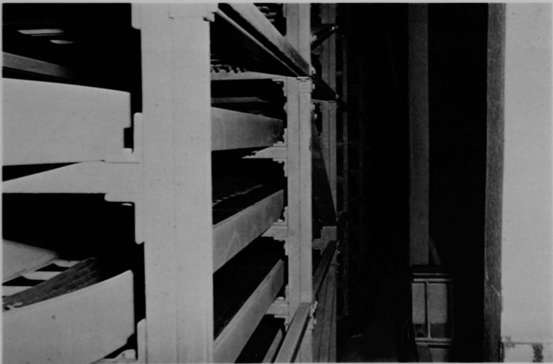
Figure 250 (6A). View south along CRDM cable trays; CRDM cables protruding in background.
