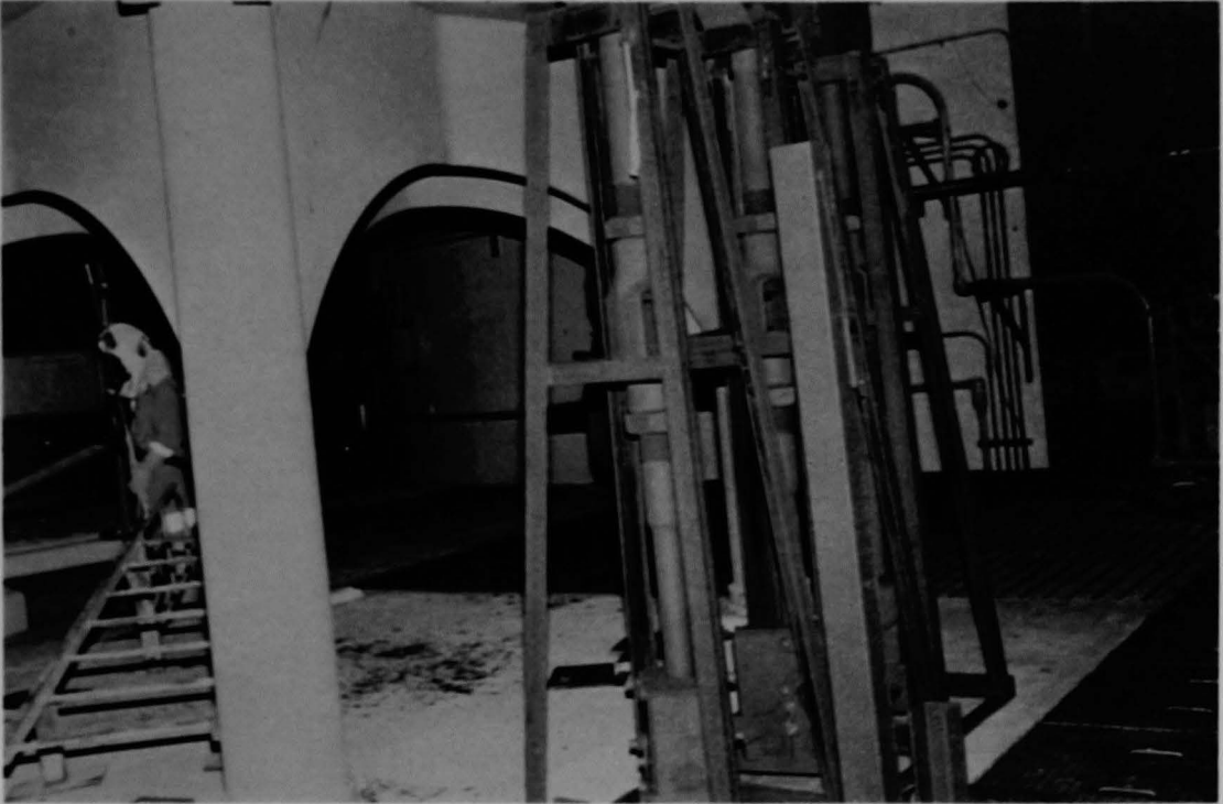
Figure 154 (2B). Internals lifting pendant.
