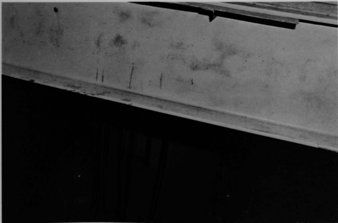
Figure 262 (2A). Reactor vessel head, fuel handling girder above
