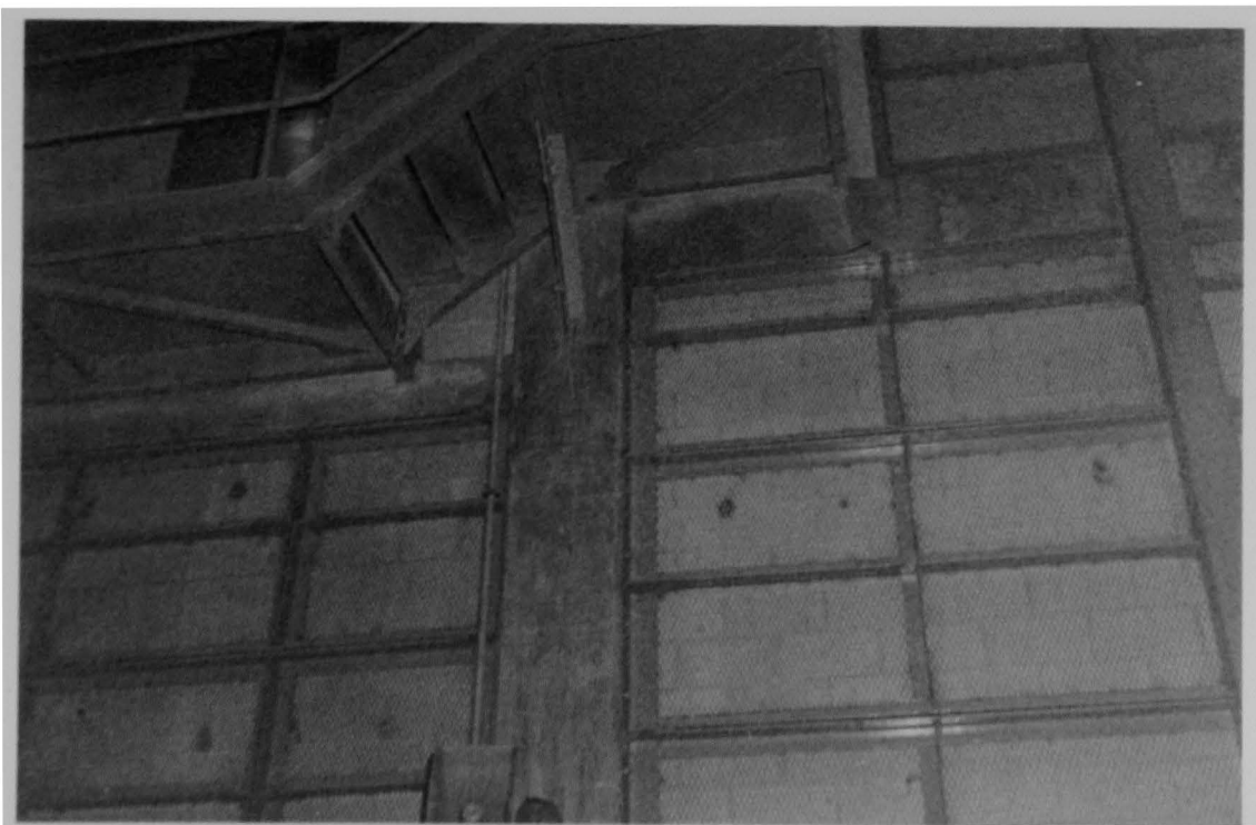
Figure 14 (6A). Platform on the enclosed elevator-stairwell, view up from elevation 305.
