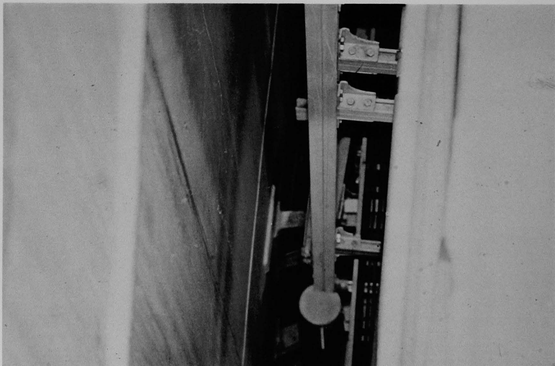
Figure 195 (4B). View down the seismic gap near the hatch over core flood tank A.
