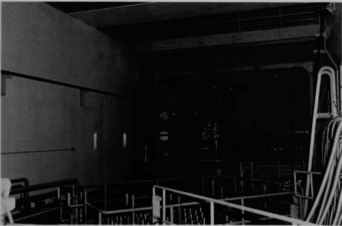
Figure 242 (2A). CRDM platform and incoming power cables, third view.
