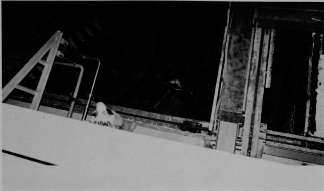
Figure 225 (5C). Reactor vessel and auxiliary fuel handling bridge from atop west D-ring; HP technician taking survey behind neutron shield tank.
