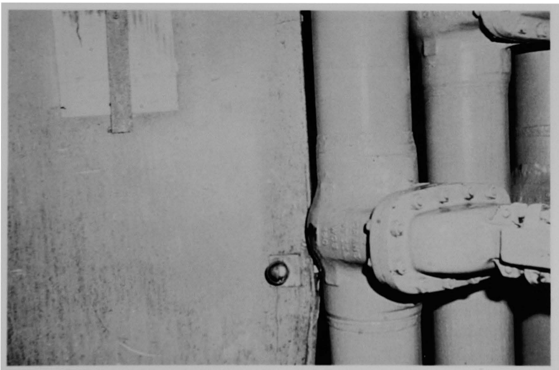
Figure 26 (1A). Close view of door to enclosed stairwell and river water piping to air cooling assembly.
