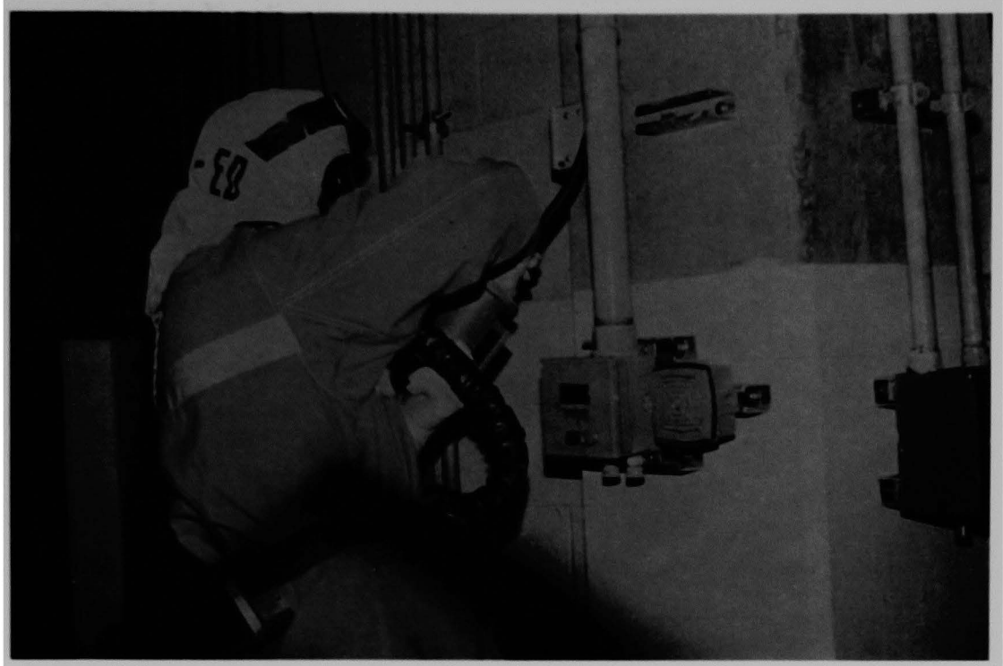
Figure 9 (2B). Technician removing HP-R-211 radiation monitor from northeast elevator wall.
