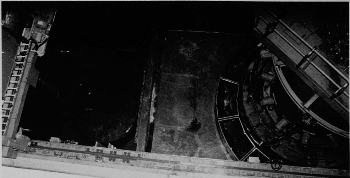
Figure 252 (5C). North end of fuel pool; main fuel handling bridge left, up ender and internals storage stand left center in deep portion of the pool.
