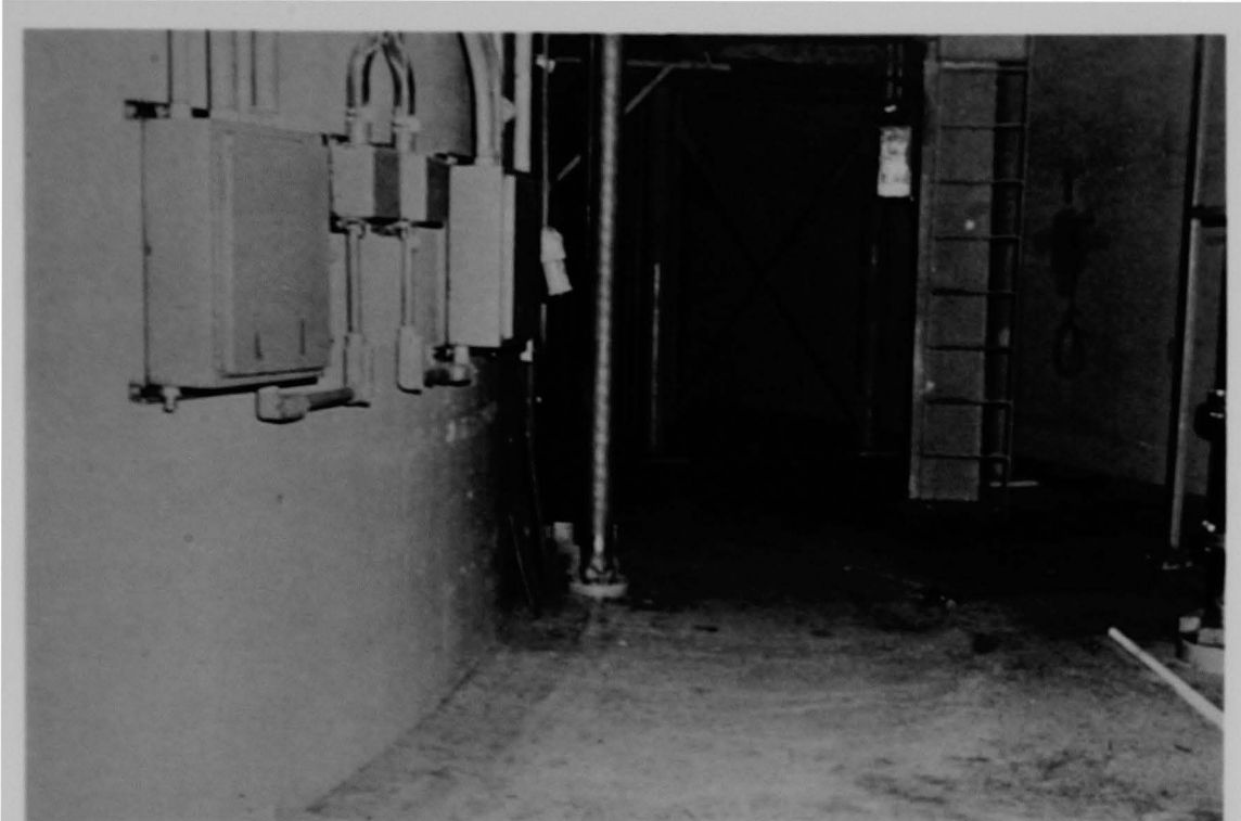
Figure 74 (1A). General view of flow area within quadrant 4 north of personnel airlock 2.
