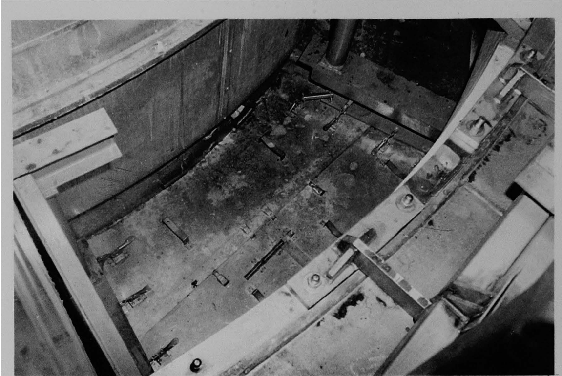
Figure 259 (5A). Close-up view under a neutron shield tank.
