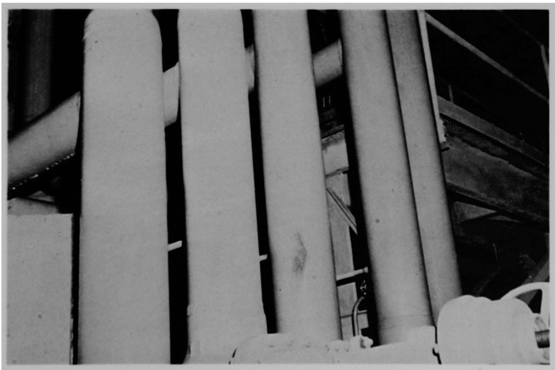
Figure 34 (1A). Close-up of river water piping associated with air coolers.
