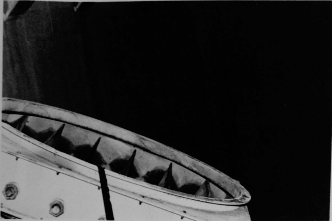
Figure 276 (5B). Top of ventilation duct near the enclosed stairwell.
