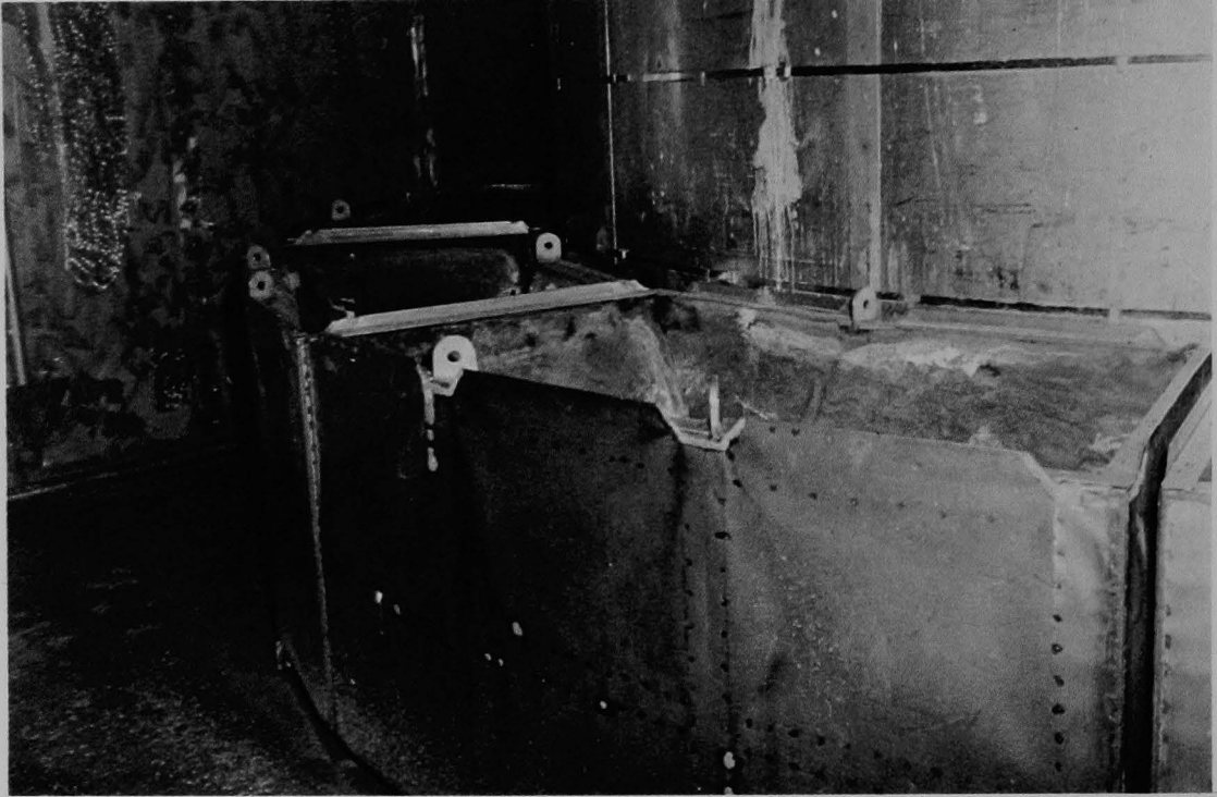
Figure 255 (5A). Base of the reactor vessel with neutron shield tanks.
