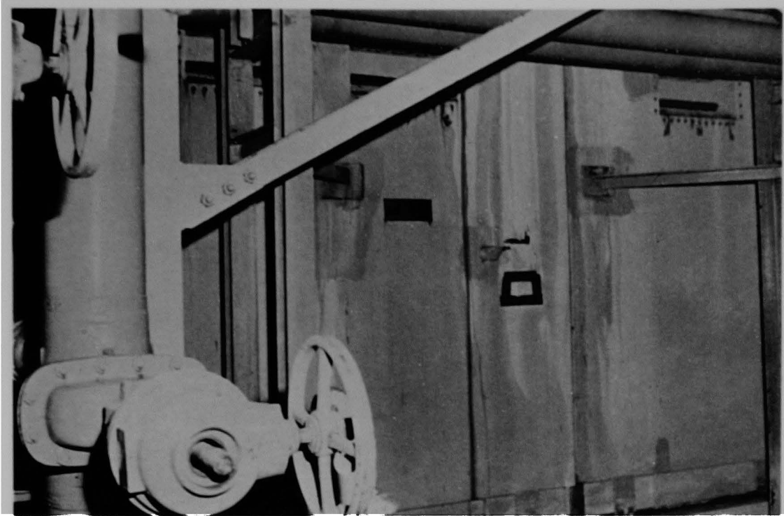
Figure 33 (1A). East units of air cooling assembly; river water piping at left.
