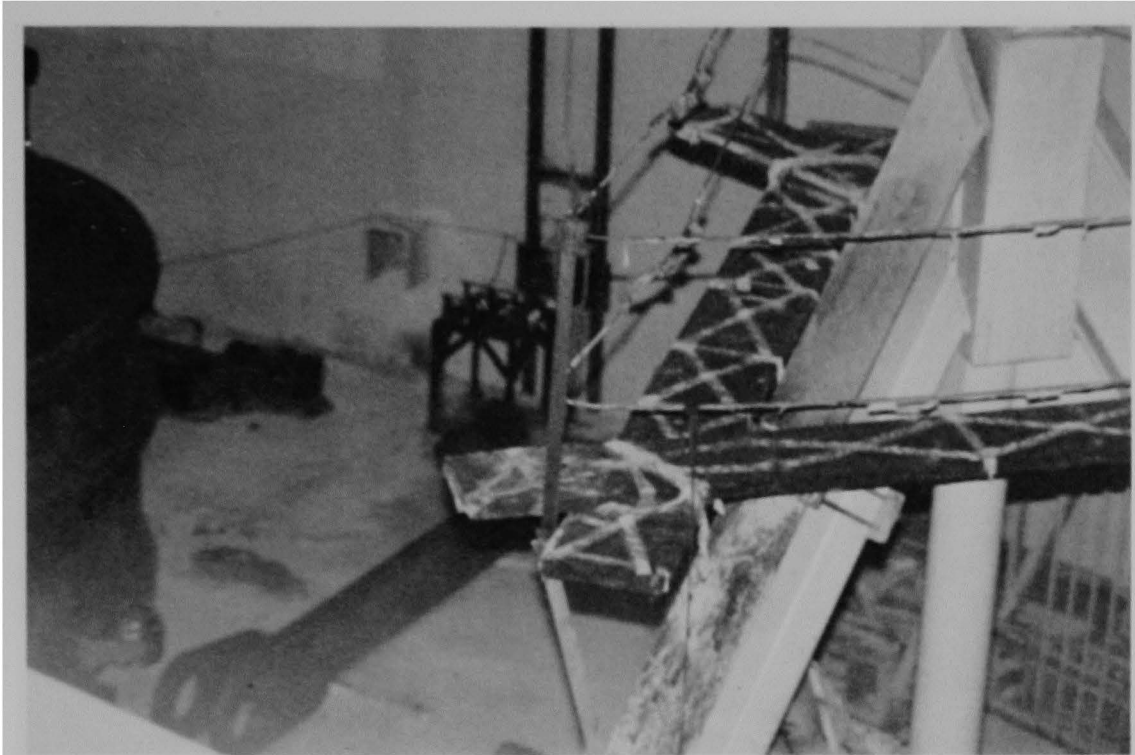
Figure 130 (4B). Scaffolding around top of head lifting rig (plastic covered); internals indexing fixture left, telephone bench background.
