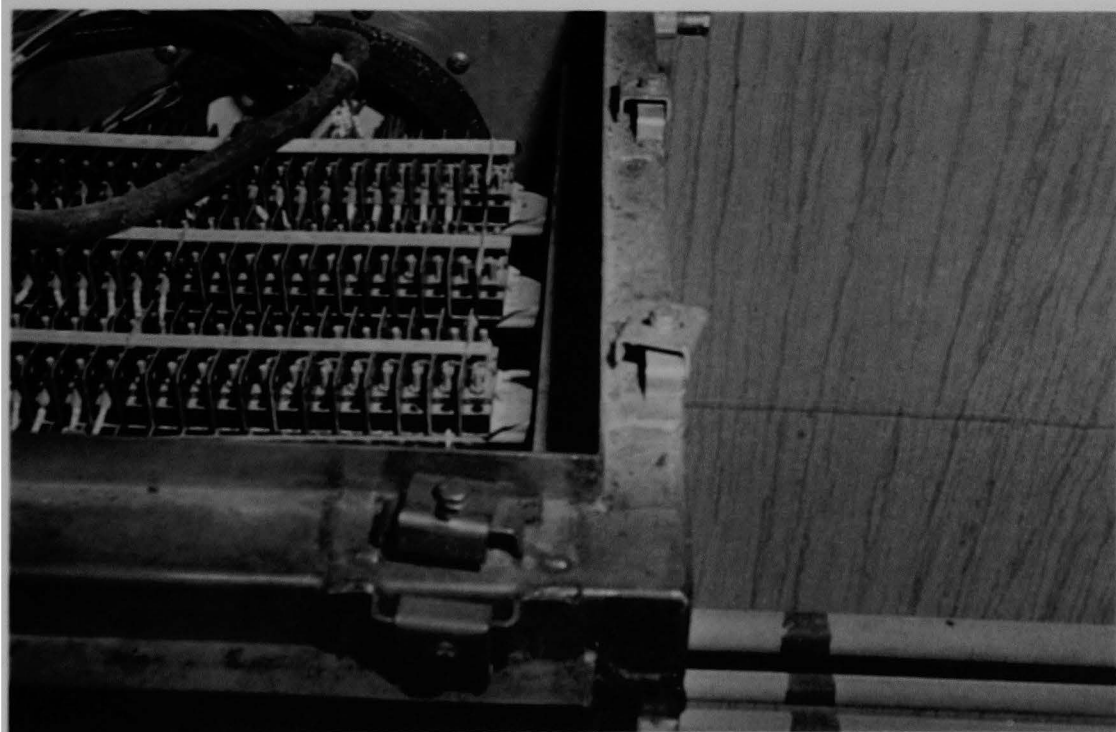
Figure 79 (6A). View of electrical penetration R-507 from above (cf. Figure 77).
