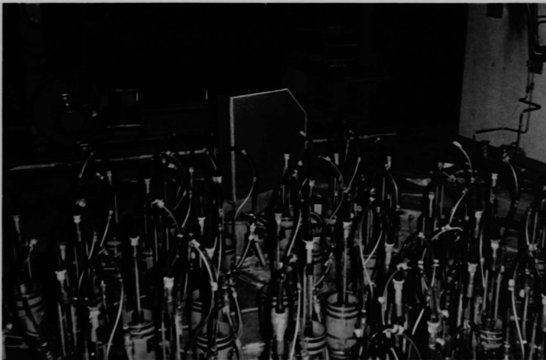
Figure 176 (4A). Incore instrumentation electrical connections, main fuel handling bridge background, closer view. (This photograph was taken to document boron crystal accumulation.)
