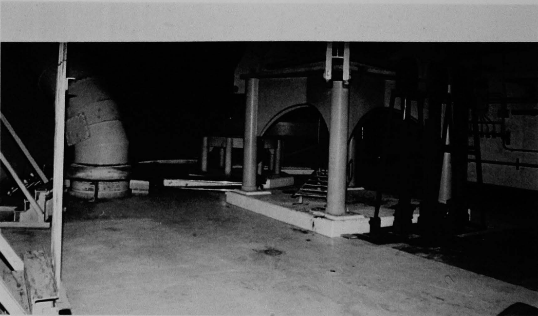
Figure 144 (2B). Panorama west from the enclosed stairwell; indexing fixture left, internals handling pendants in their storage stands and reactor coolant pump with vessel head and internals center.
