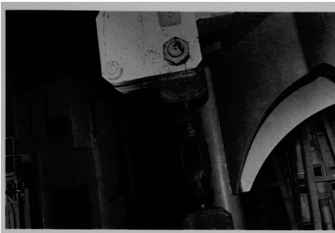
Figure 170 (2B). Extension pendant handing from the handling fixture atop the pump stand.
