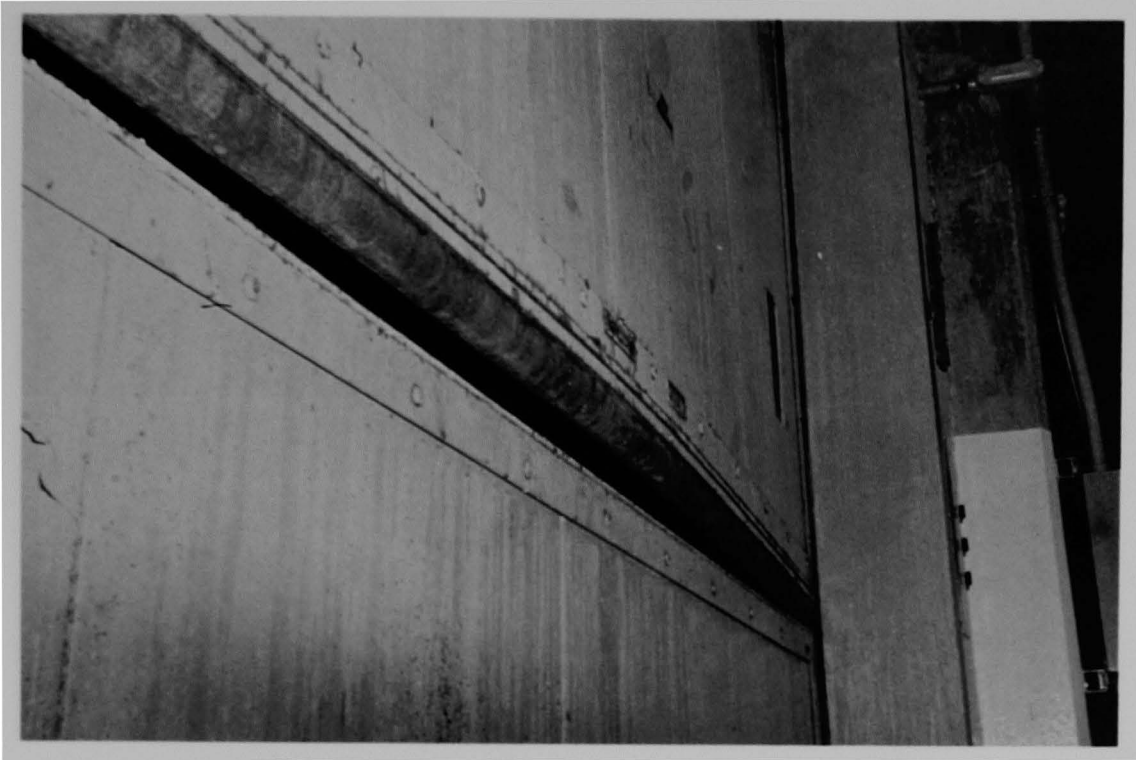
Figure 13 (6A). Close-up of gap in elevator door.
