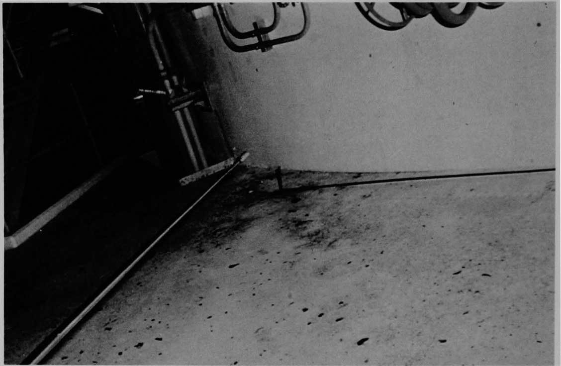
Figure 58 (1A). Broken glass on floor (teletector probe appearing from left corner of photograph).
