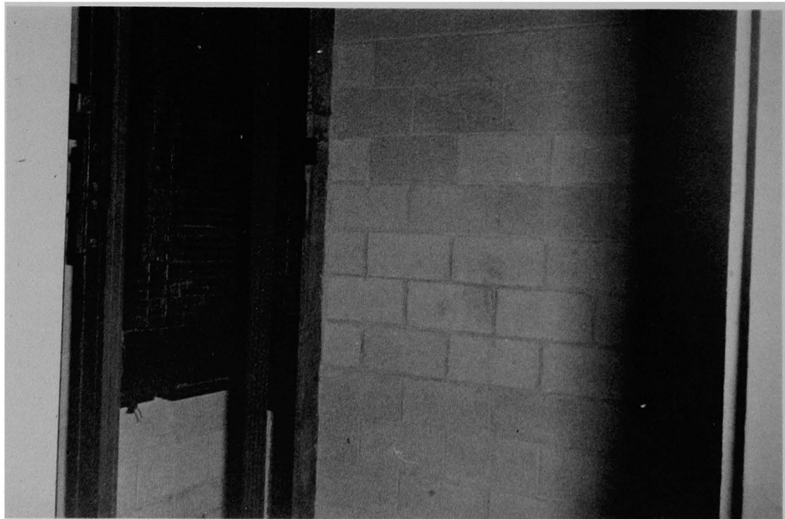
Figure 16 (6A). Inside of the elevator shaft, view through door shown in Figure 15.
