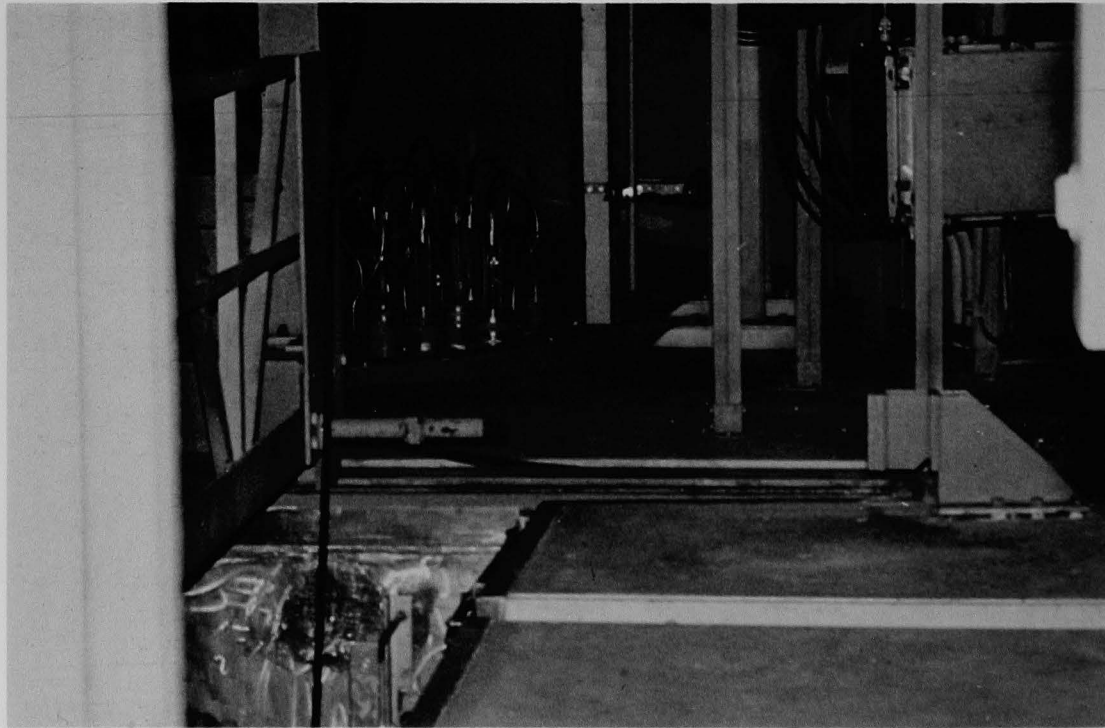
Figure 182 (4B). North end of the fuel pool; incore seal table background, main fuel handling bridge left.
