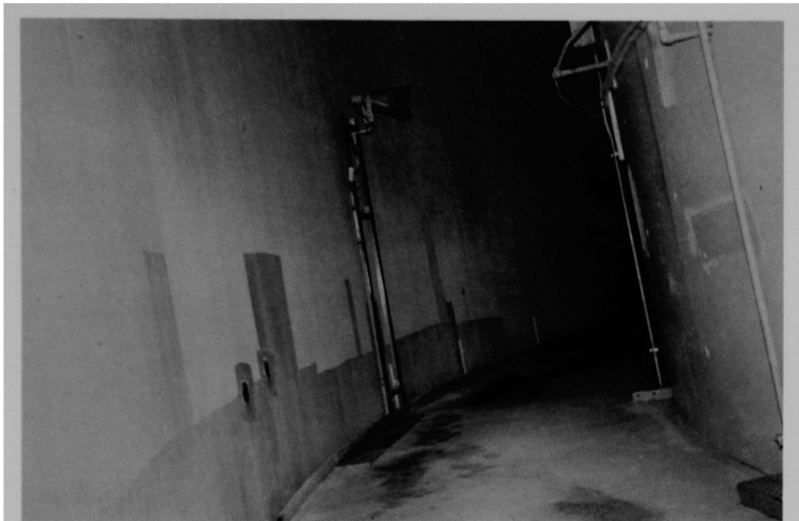
Figure 171 (2B). Area just north of the open stairway.
