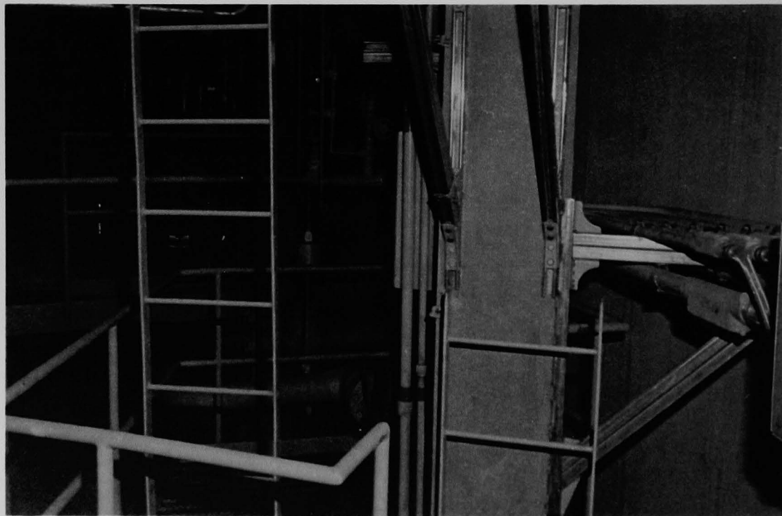
Figure 85 (6A). View north from scaffolding erected at overhead piping, near core flood tank A.
