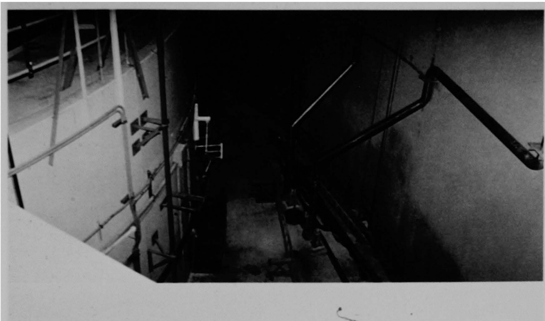
Figure 184 (5C). East side of containment from atop the elevator. (Note that the building spray lines turn up at right.)
