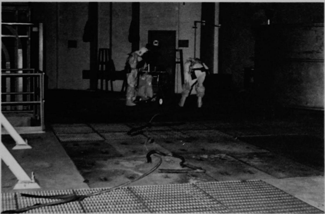
Figure 167 (4 ). Southeast across the operating deck toward the enclosed stairwell; technicians are working with video camera.
