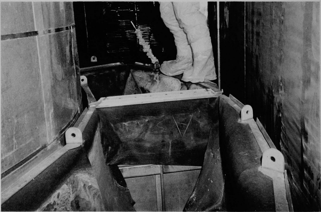
Figure 256 (5A). View inside of neutron shield tank (technician on shield tank to gain access to the north side of the reactor vessel).
