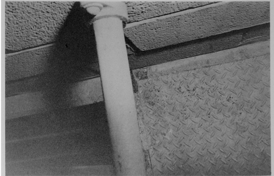
Figure 29 (6A). Close-up of landing within the enclosed stairwell.
