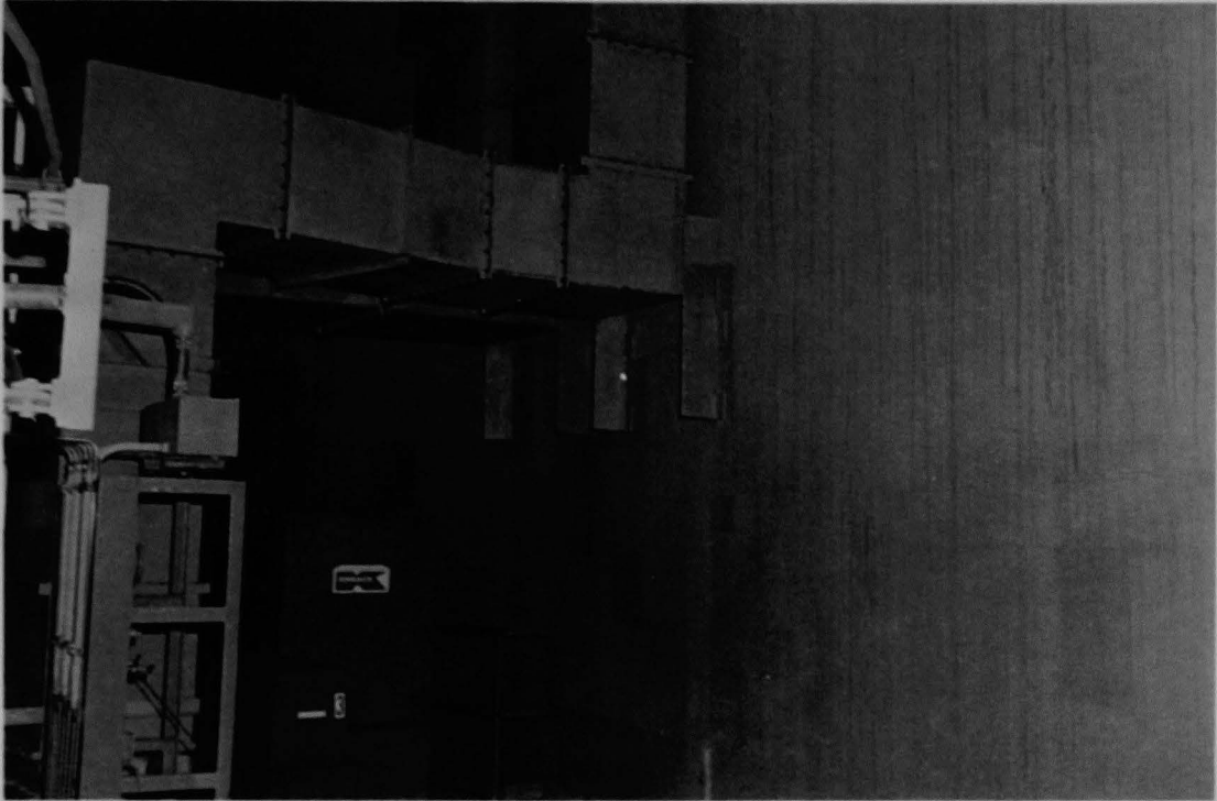
Figure 192 (6A). Purge ducting and tool boxes (cf. Figure 211).
