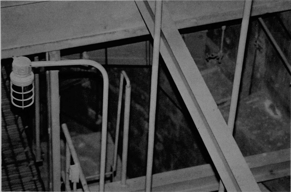
Figure 211 (4B). Inside D-ring A near the pressurizer.
