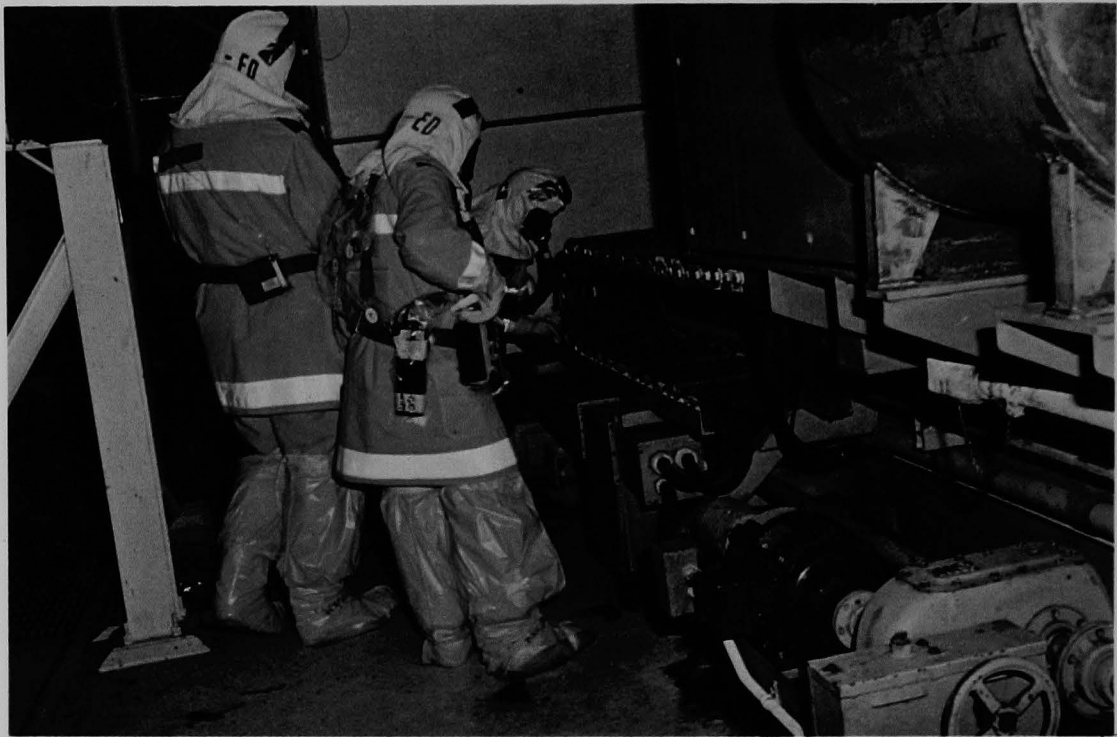
Figure 223 (2A). Power track and bridge motor of auxiliary fuel handling bridge, view from southeast, with HP technicians.
