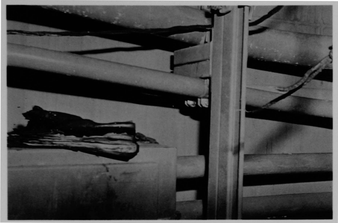
Figure 200 (6A). Charred manual lying on top of electrical box.
