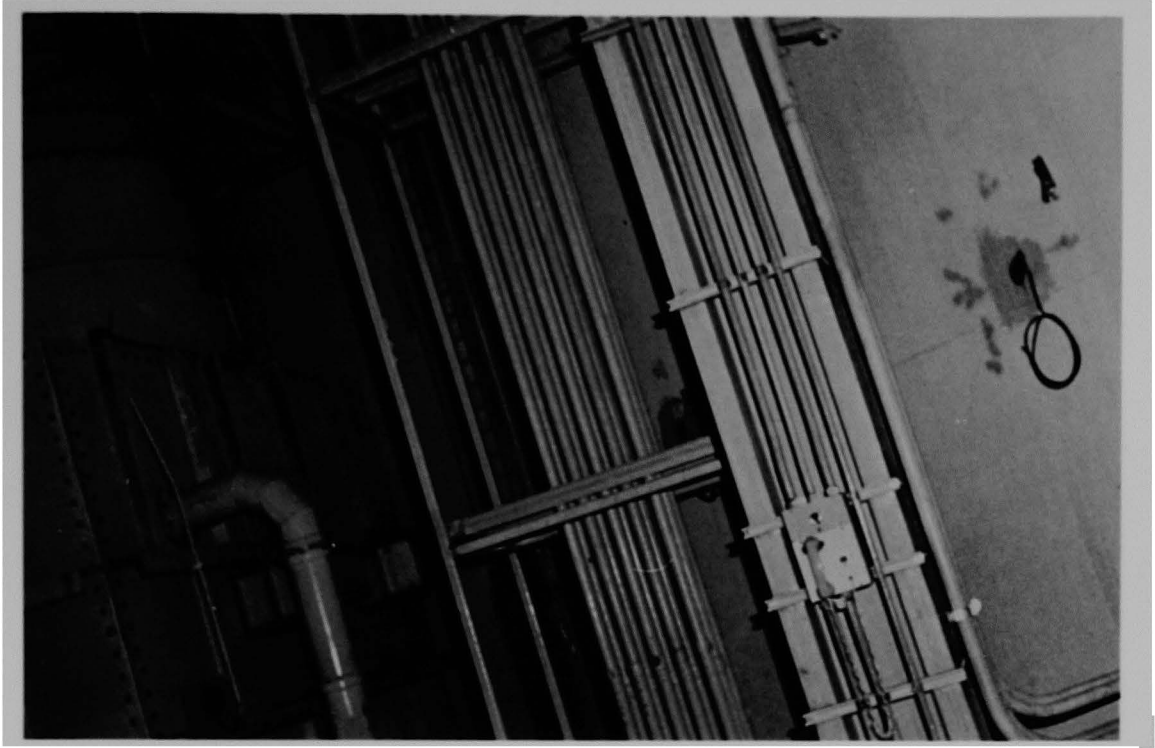
Figure 48 (1A). Conduit runs, plenum at west end of air cooling assembly left.
