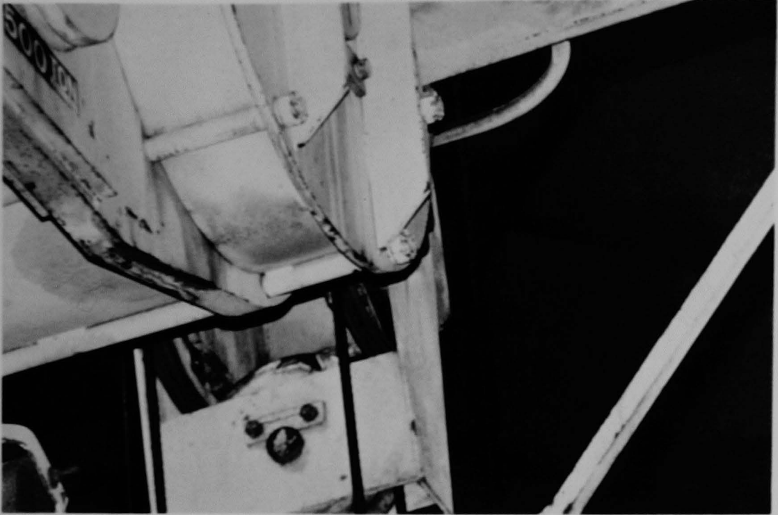
Figure 296 (5B). Main hook of the polar crane, fifth view.
