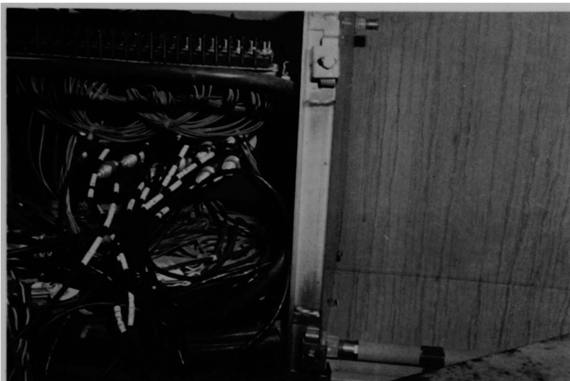
Figure 78 (6A). Right frontside of electrical penetration R-507 (cf. Figure 77).
