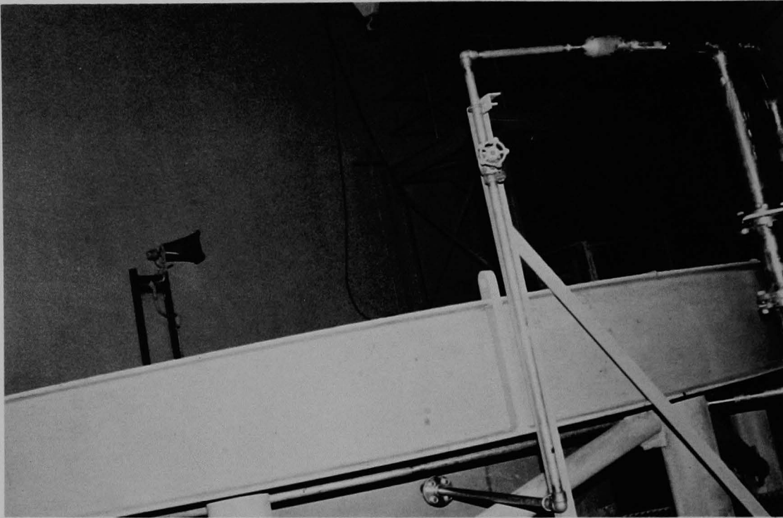
Figure 160 (2B). Close-up of the reactor vessel head storage stand; open stairway in background.
