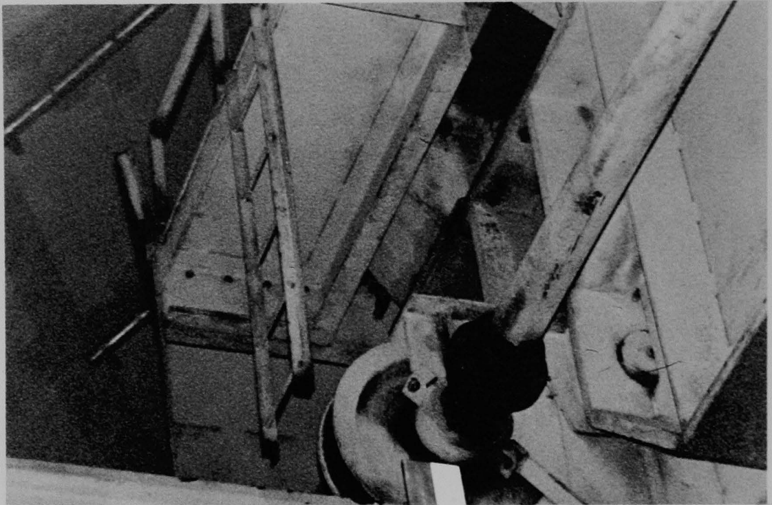
Figure 274 (5B). Trolley and one of its wheels.
