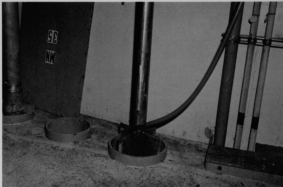
Figure 81 (6A). Floor penetrations 210, 211 and 211 on east side of D-ring wall.
