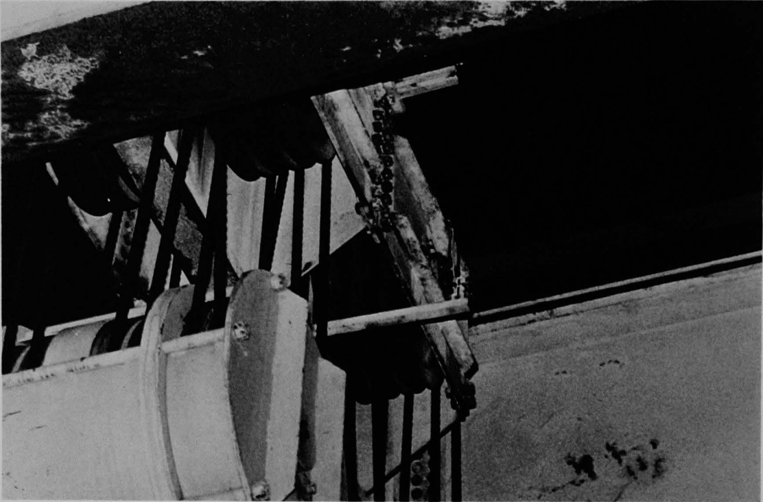
Figure 298 (5B). Cable drum and the main block of the trolley on the polar crane, second view.
