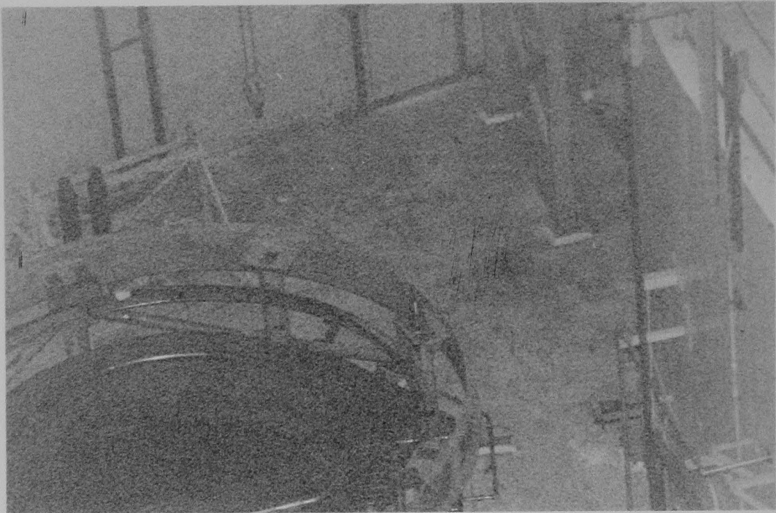
Figure 156 (5B). Reactor vessel head storage stand.
