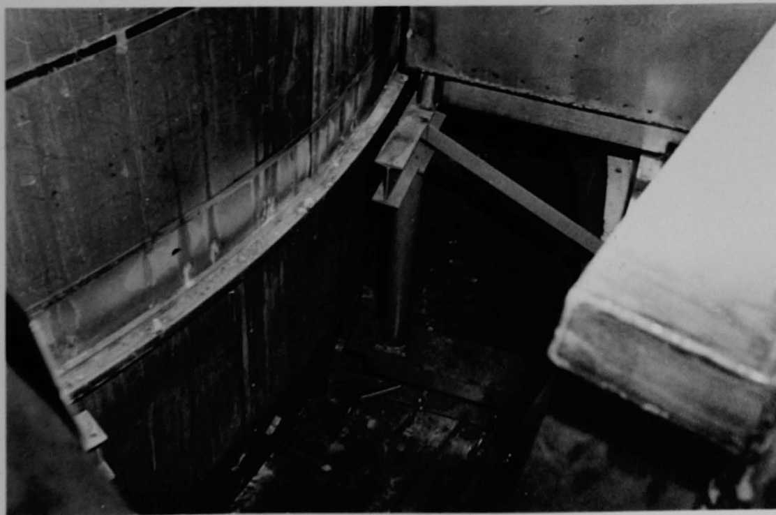
Figure 258 (5A). Second view underneath a neutron shield tank.
