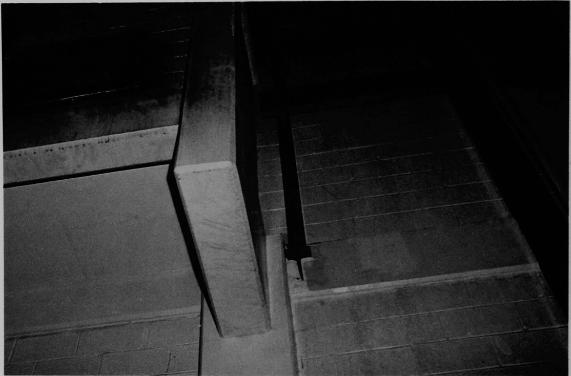
Figure 99 (4A). Ventilation grill into the elevator shaft motor room (see Figure 97, upper left center).
