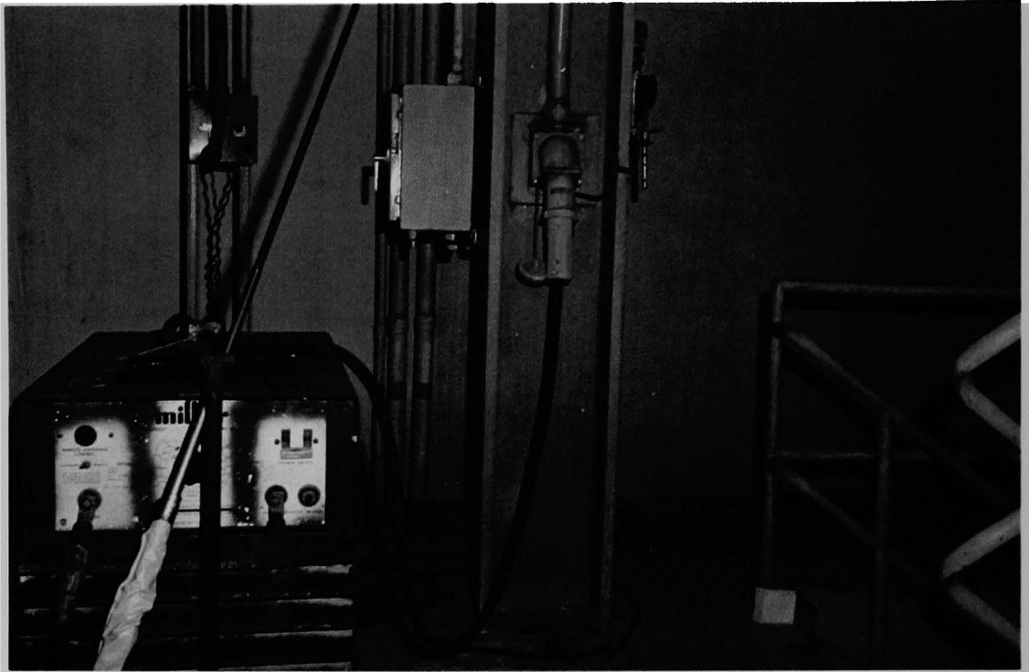
Figure 54 (2A). Rusted welding box; Gai-tronic phone in background, open stairway at right.
