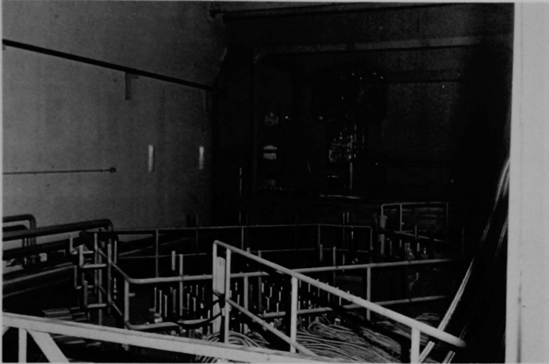
Figure 241 (2A). Control rod drive mechanism platform and power cables; main fuel handling bridge background, second view.
