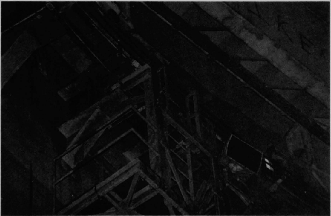
Figure 269 (5B). Close-up of the access platform to the polar crane.
