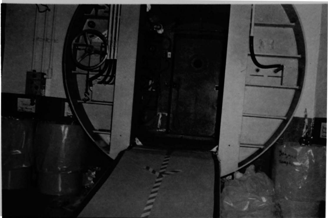
Figure 1 (4A). Anteroom entry ramp into personnel air lock 2.
